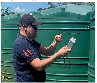
Installing the level sensor and LoRa modem
