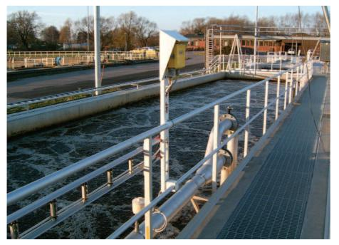
Compressed air is typically used to provide the air to the aeration basins. Controlling the proper amount of air that is released into the aeration basins is essential because it controls the growth of microorganisms that treat the wastewater. Flow meters are typically installed in the aeration system piping to measure the amount of air flow and the meters' analog or digital outputs run to the control system.
