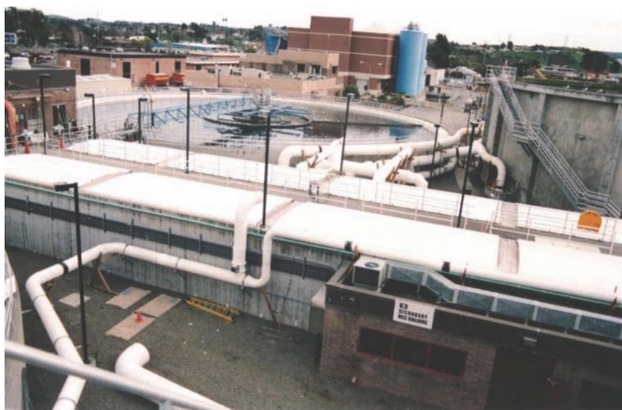
Vallejo's new retractable, structurally-supported geomembrane cover system – designed, engineered and built by GTI – consists of a composite sheet of high-strength, UV-protected, coated fabric tensioned across a series of low-profile aluminum arches which span the tank's opening. Intermediate aluminum walkways spanning the tank are used to divide the fabric cover sections into appropriate lengths for easy retractability.
