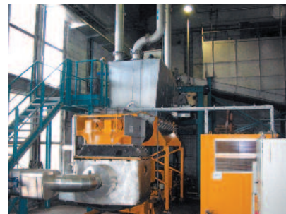
Fig. 3 KOS 25100 with Hydraulic power pack and twin-screw auger feed device, conveying biomass to the fermentation tank (Biogas plant in Leonberg, Germany).
