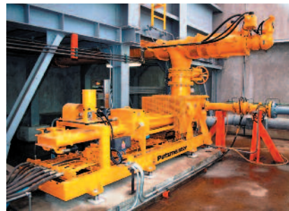
Fig. 2 At the Siam City Cement plant (Thailand), this Putzmeister high-density solid pump conveys substitute fuels (i.e. sludges of varying consistency) in incinerators which are up to 150 m away
