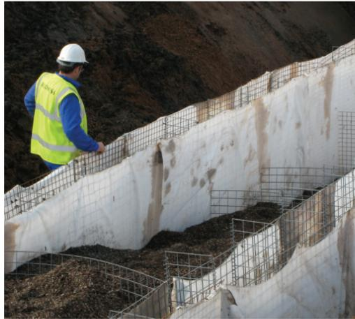
The NITRABAR project has been underway since December 2005 and in order to test the technology a demonstration site has been established at the Ecos Millennium Environmental Centre, Ballymena in Northern Ireland where the NITRABAR system is being continuously monitored to prove its performance under varying ground conditions and nitrate fluxes.
