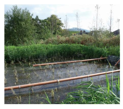
In FBA $^{\text{m}}$  systems, a network of aeration pipes are laid below the gravel matrix. Air is then forced through these pipes enabling a constant flow to percolate through the system thereby increasing the oxygen availability. This boosts treatment capability by up to 15 times greater than that of a traditional passive reed bed. This also means that FBA $^{\text{m}}$  reed bed treatment systems can treat heavier loads in smaller footprints than existing systems.
