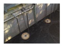
Designed to cater for a population of approximately 850, Iseltwald wastewater treatment plant in Brienz, Switzerland, consists of a 10m deep activated sludge tank and a tank for the aerobic treatment of primary sludge. A total of five Tsurumi FHP pumps are in use at the plant, four are situated in the activated sludge tank, which measures 6% solidity, and one in the aerobic
