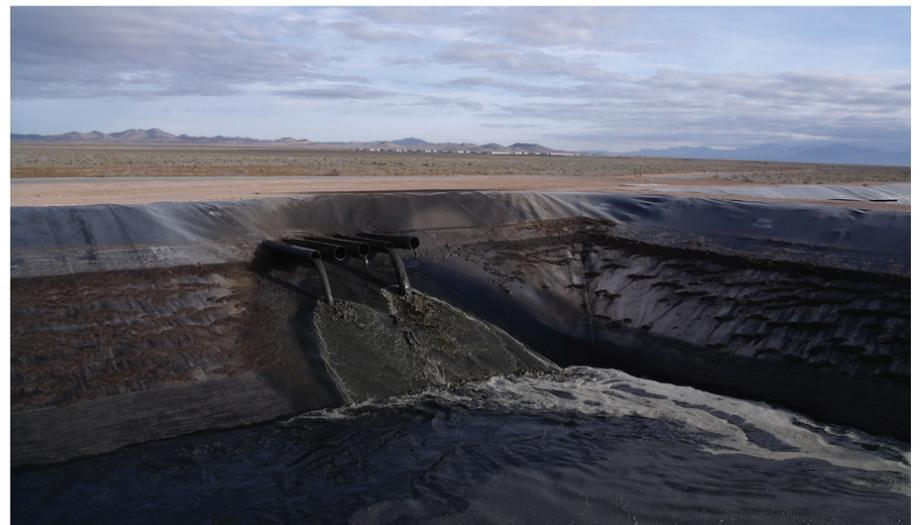
Fig. 1 Liquid effluent is pumped from finishing barns to a one million gallon influent basin.
