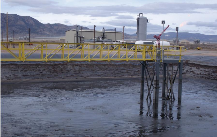
Fig. 3. KSB Amaprop hybrid submersible agitator with self-cleaning propeller is mounted on a guide mast located on the bridge extending above the surface of the basin.
