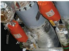
and increase costs. A steam trap is the most important link in the condensate loop, because it connects steam usage with the condensate return.
