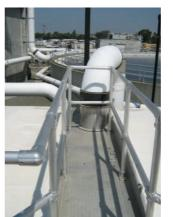
The material can withstand temperatures to minus 30 degrees F. This cover has exceptional seam strength, extreme puncture and tear resistance, low thermal expansion and contraction properties, a wide range of chemical resistance, high flexibility, and dimensional stability under high loads and temperature fluctuations, making it ideal for wastewater cover applications.
