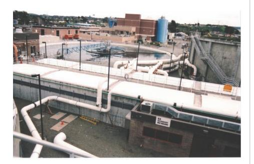
Vallejo's new retractable, structurally-supported geomembrane cover system – designed, engineered and built by GTI – consists of a composite sheet of high-strength, UV-protected, coated fabric tensioned across a series of low-profile aluminum arches which span the tank's opening. Intermediate aluminum walkways spanning the tank are used to divide the fabric cover sections into appropriate lengths for easy retractability.
