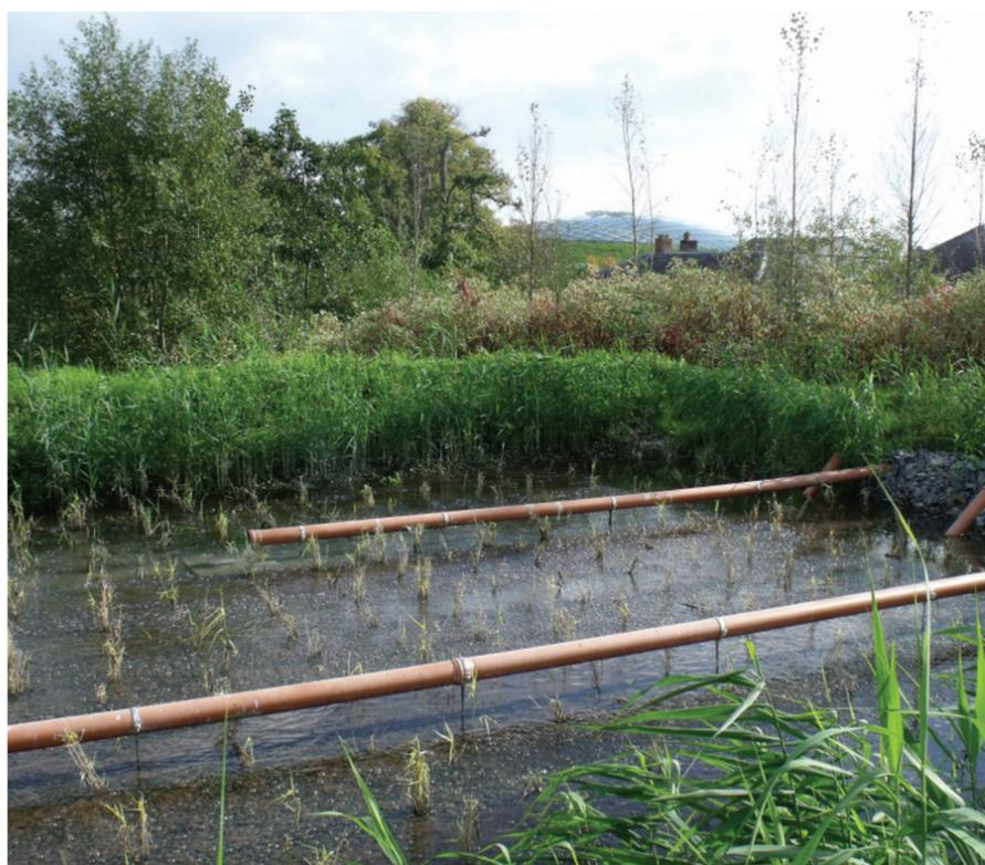
In FBA™ systems, a network of aeration pipes are laid below the gravel matrix. Air is then forced through these pipes enabling a constant flow to percolate through the system thereby increasing the oxygen availability. This boosts treatment capability by up to 15 times greater than that of a traditional passive reed bed. This also means that FBA™ reed bed treatment systems can treat heavier loads in smaller footprints than existing systems.
